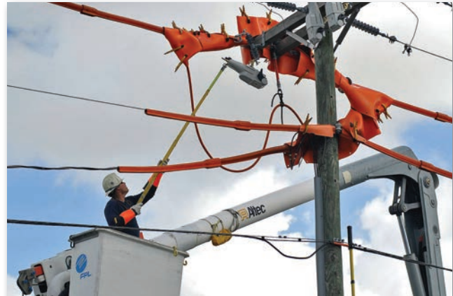
FPL team installs TripSaver II reclosers.
