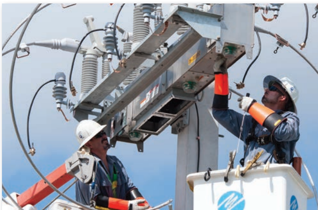
An IntelliRupter fault interrupter being installed.
