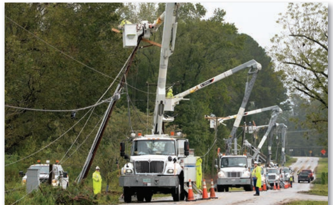
FPL team restores power after the hurricane.
