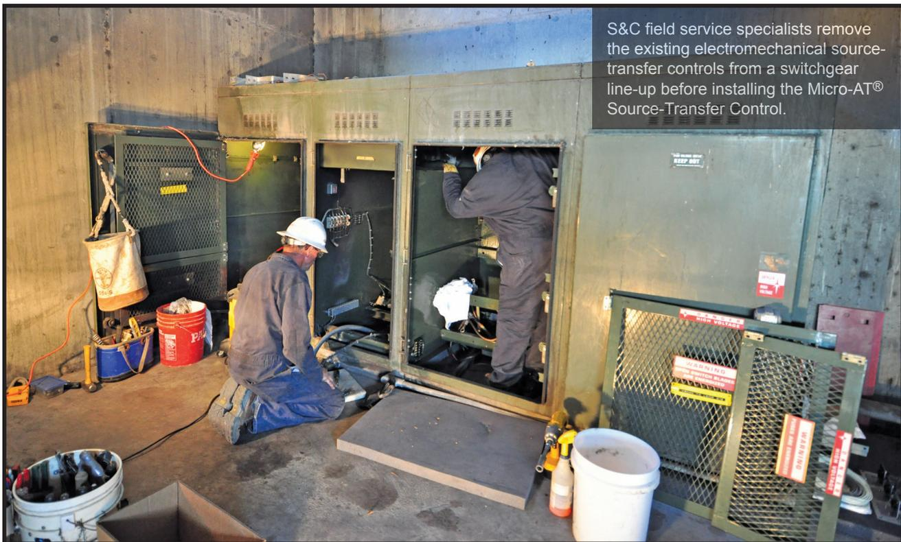
S&C field service specialists remove the existing electromechanical source-transfer controls from a switchgear line-up before installing the Micro-AT® Source-Transfer Control.
